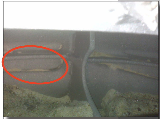
Figure 3: Customer C who ran his REMco unit empty that resulted in exposure and erosion of the rock shelf.
